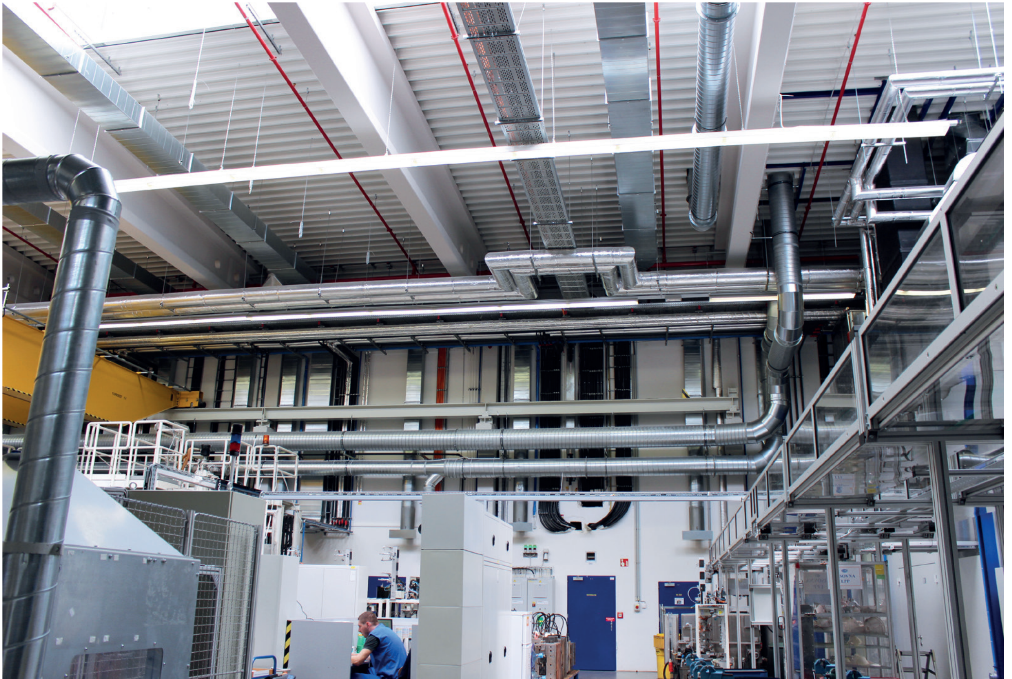
Exhausting the workplaces LPP in the hall B8 HELLA Autotechnik, Mohelnice ; HELLA; Czech Republic; 2013
