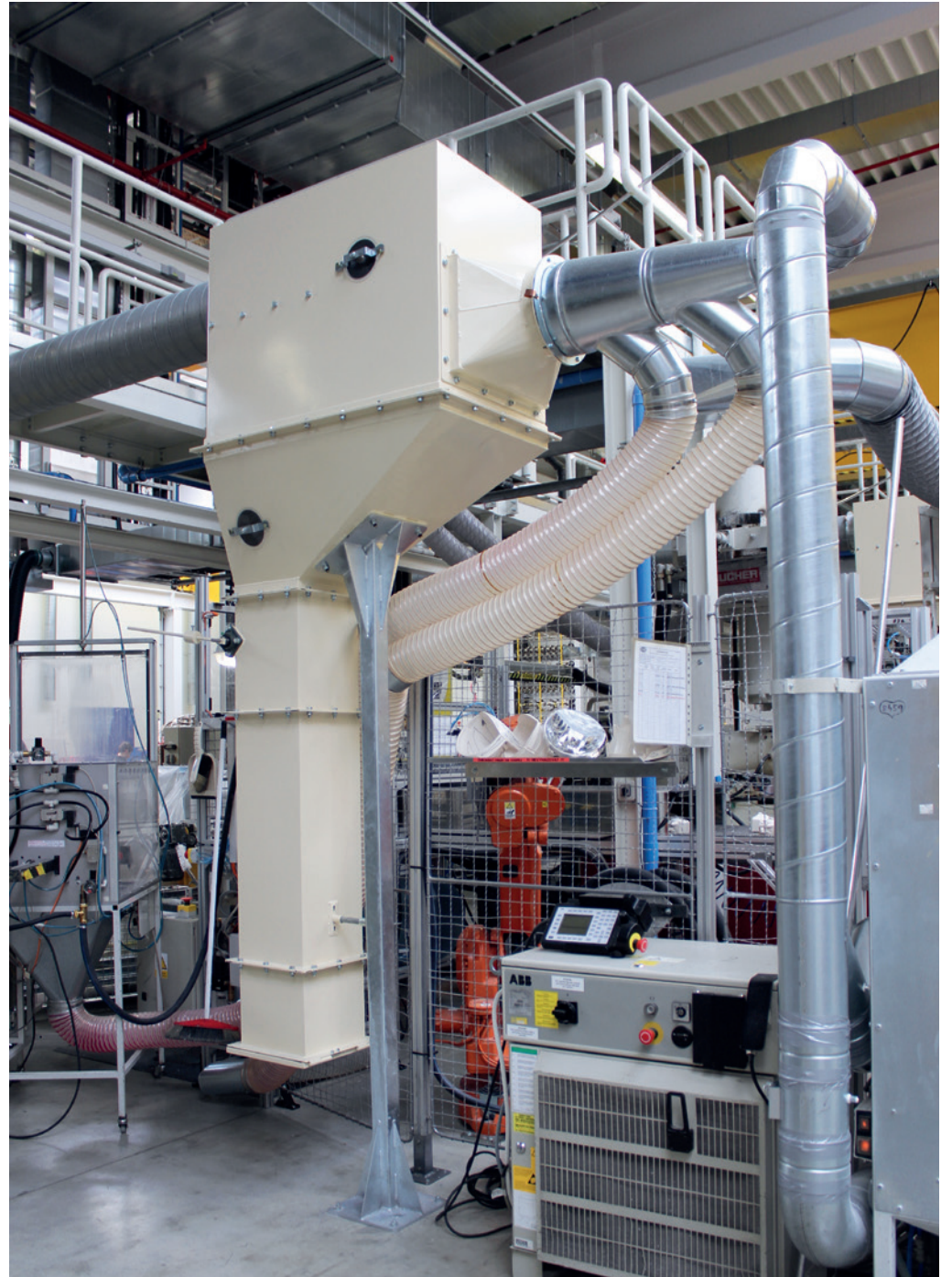
Exhausting the workplaces LPP in the hall B8 HELLA Autotechnik, Mohelnice ; HELLA; Czech Republic; 2013
