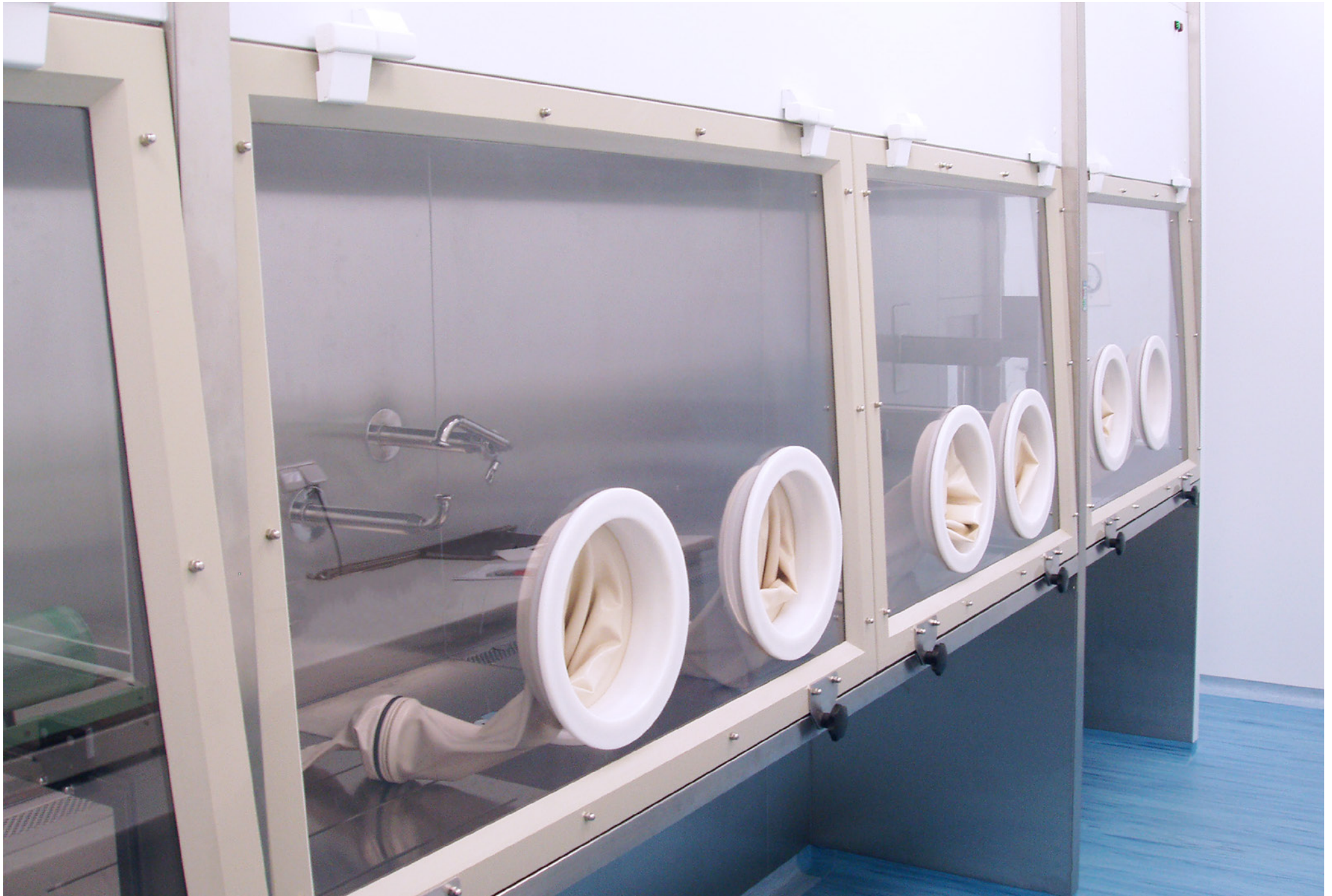
Completion of CONTIPRO a.s. Facilities – Stage II; Contipro a.s.; Ústí nad Orlicí, Czech Republic; 2006
