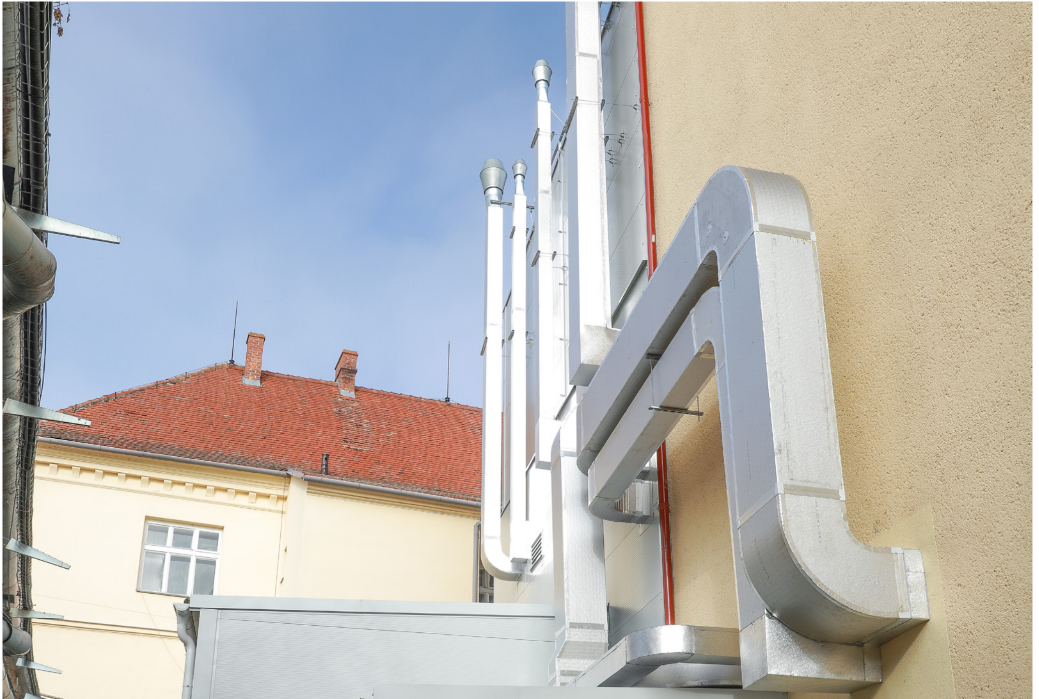
Construction Work and Extension of Building No. 3 for the Production of Hormonal Preparations; Bioveta, a.s.; Ivanovice na Hané, Czech Republic; 2020
